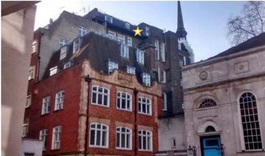
VIEW OF THE REAR OF 38 LUDGATE HILL
